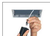
Connect luminaire to electrical power supply
